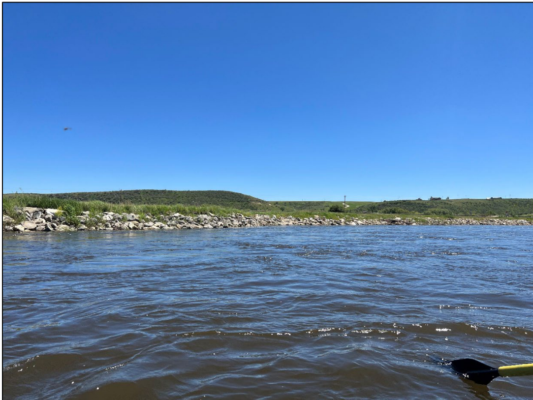
Figure A-4. Bank armoring with large boulders.
