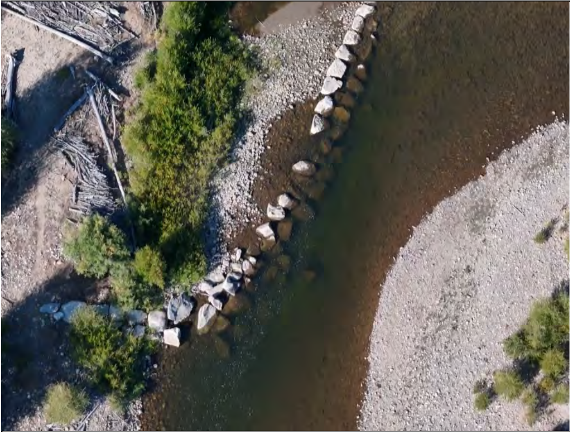
Figure A-3. Grade control structure (j-hook) in riverscape 10
