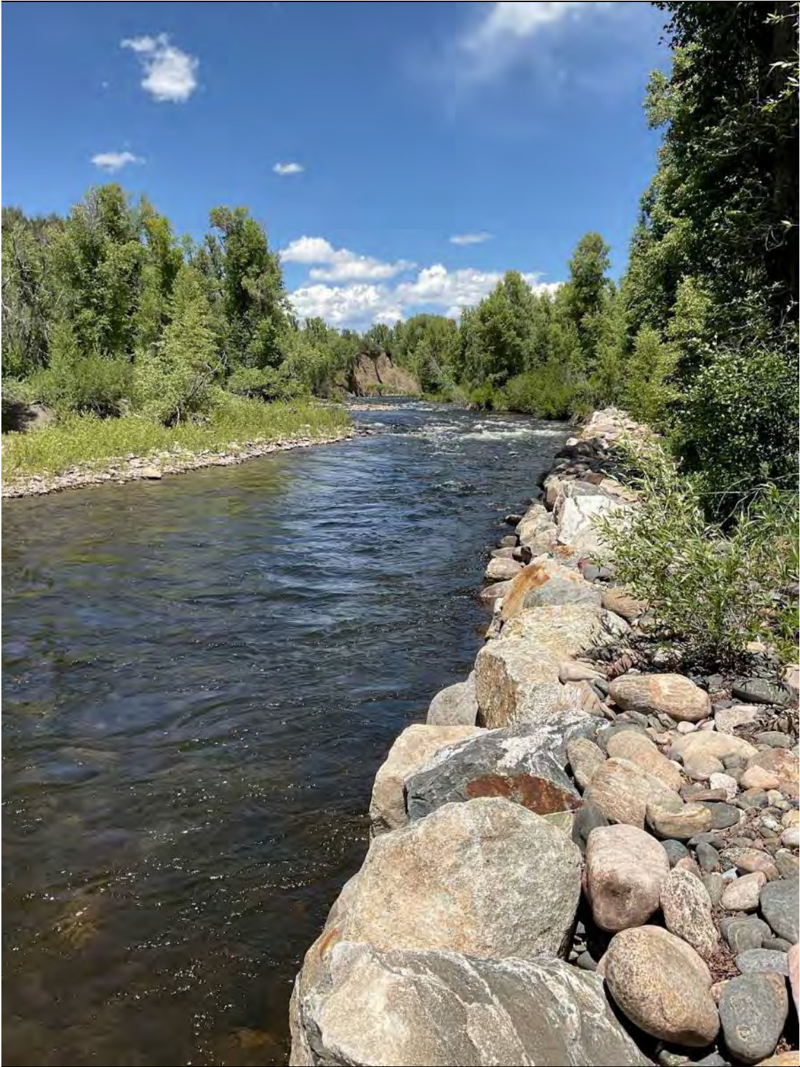
Figure A-11. Bank armoring in riverscape 9
