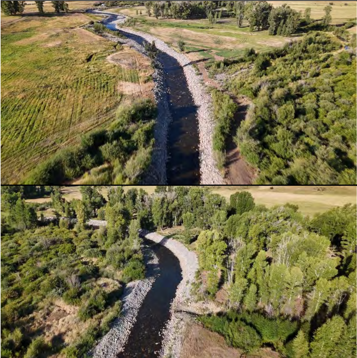
Figure A-8. Extensive armoring on both sides of the river in riverscape 9, looking downstream
