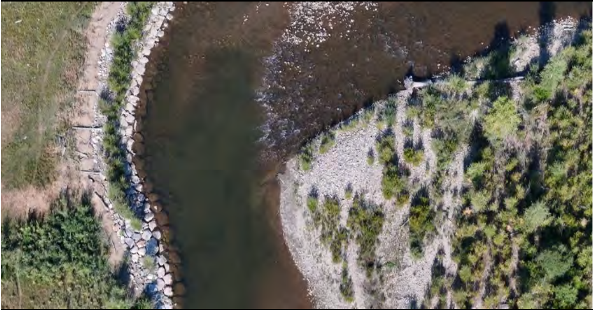
Figure A-31. Example of modified riverbank and floodplain (left) opposite a relatively intact, natural channel and floodplain (right) in riverscape 10
