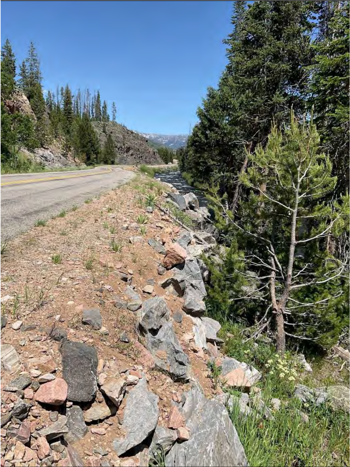
Figure A-13. Bank armoring along Seedhouse Road in riverscape 8
