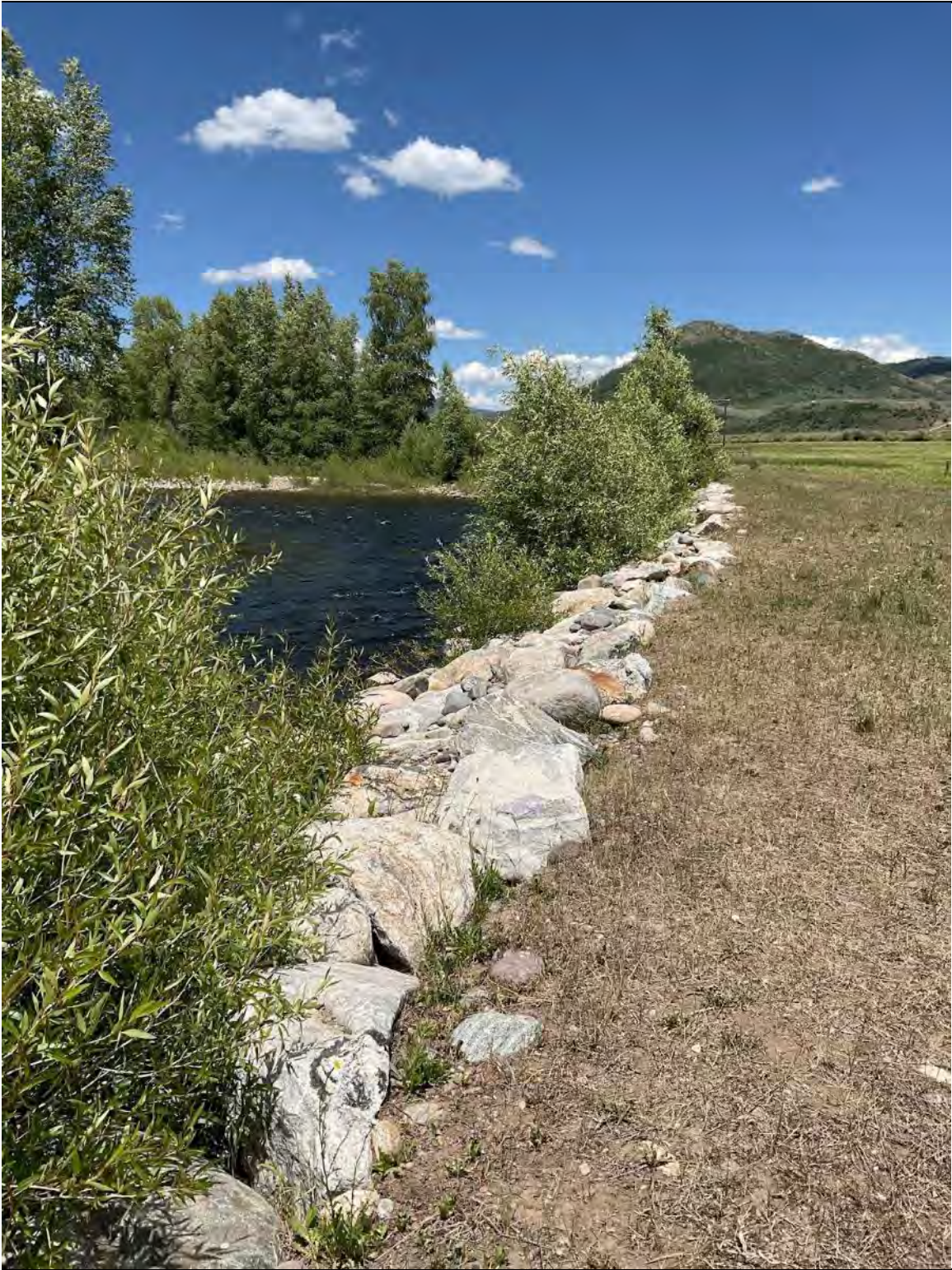
Figure A-12. Bank armoring in riverscape 10
