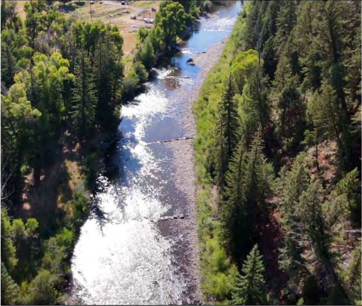
Figure A-2. Several grade control structures (cross vanes) in riverscape 11 (looking downstream)
