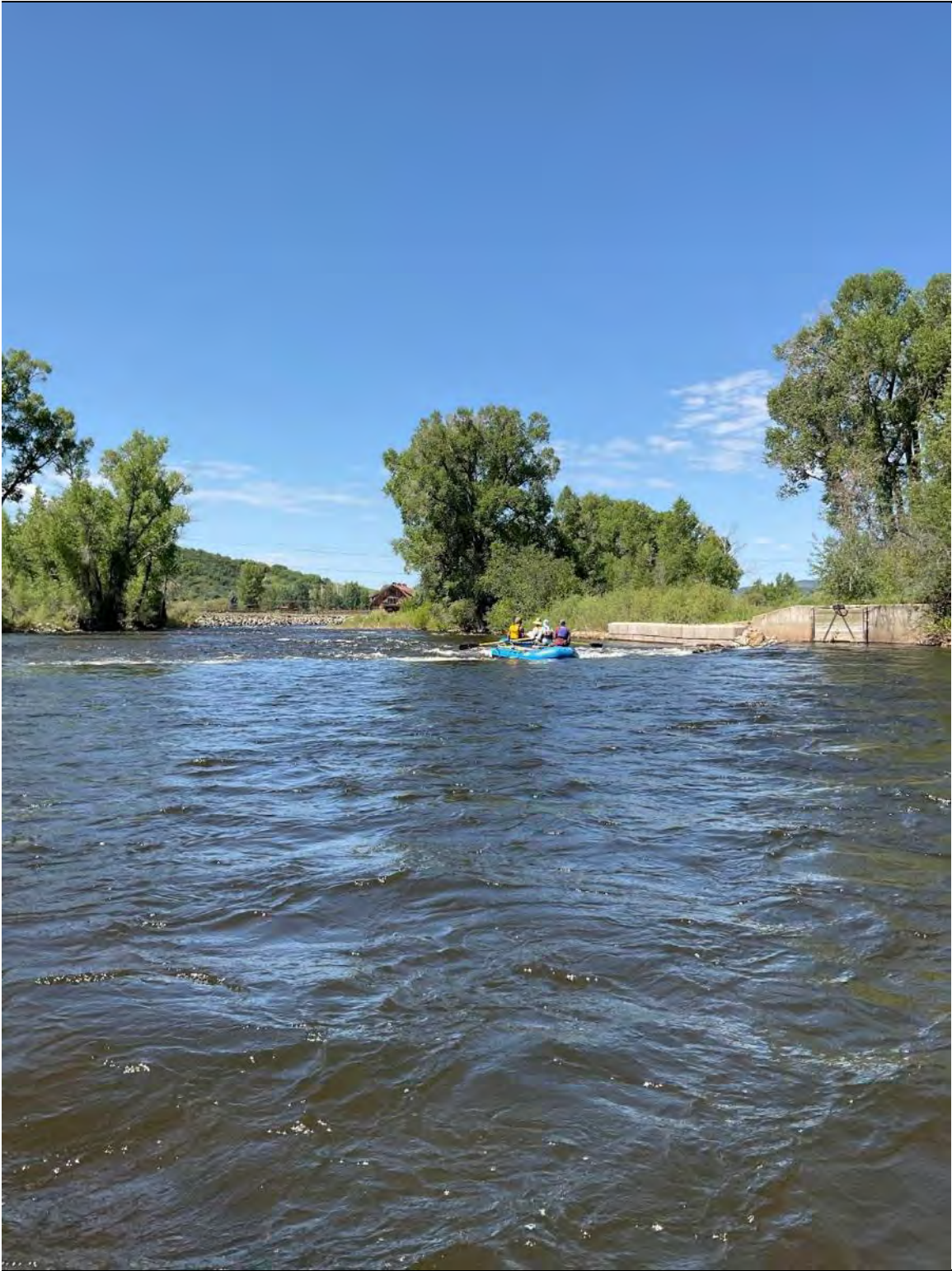
Figure A-4. Diversion structure (“push-up” dam & intake/headgate) in riverscape 12
