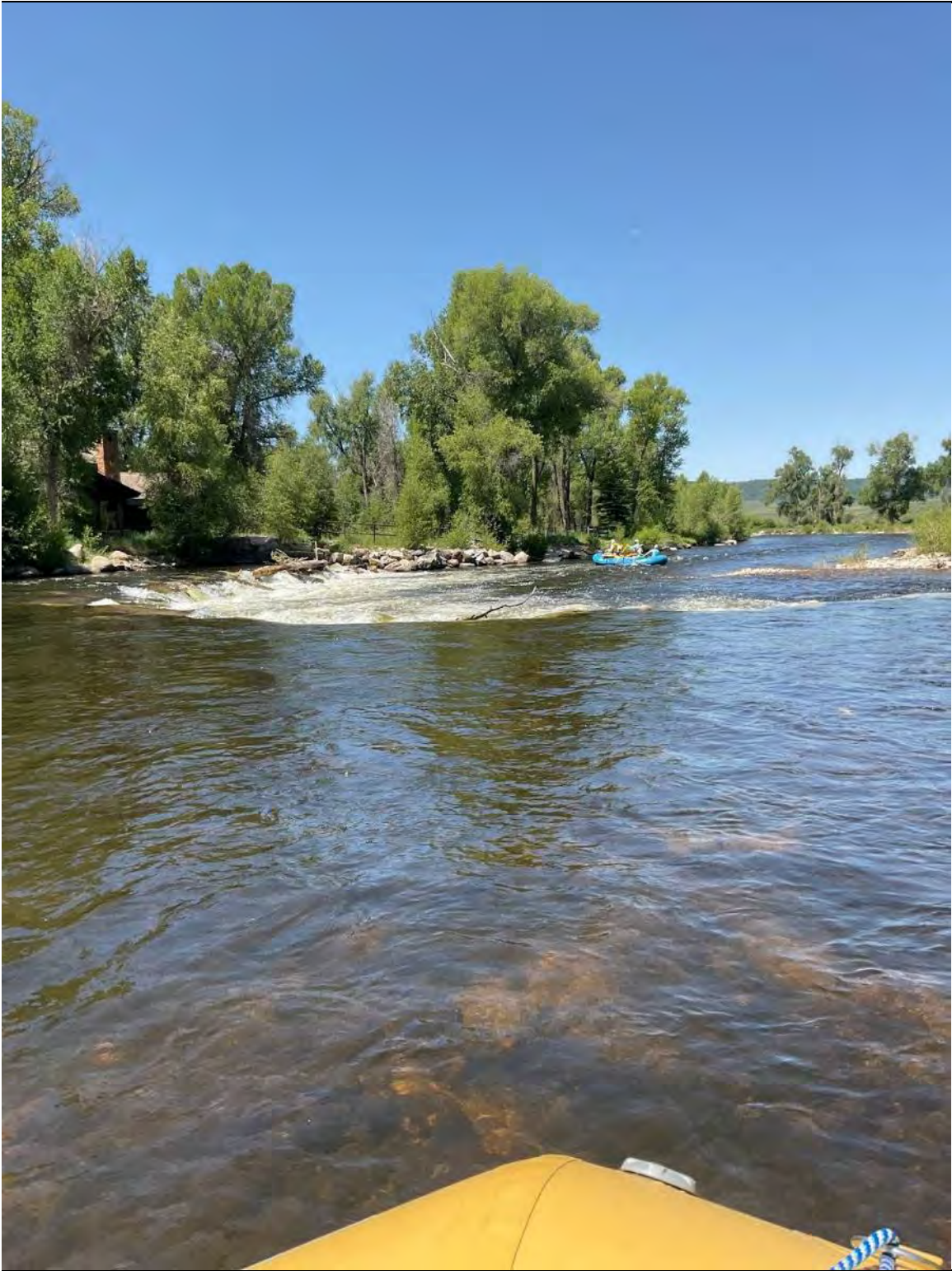
Figure A-1. Large grade control structure (cross vane) in riverscape 12 (looking downstream)
