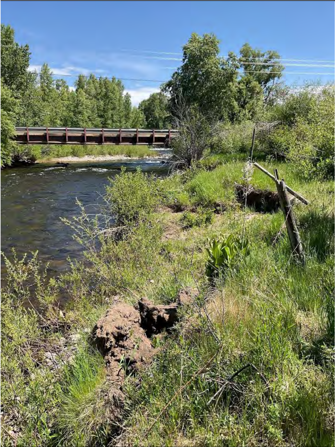
Figure A-6. County road bridge in riverscape 9
